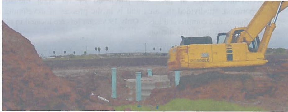
Source: Design Services, Inc. 2007 Construction of wastewater lift-station
